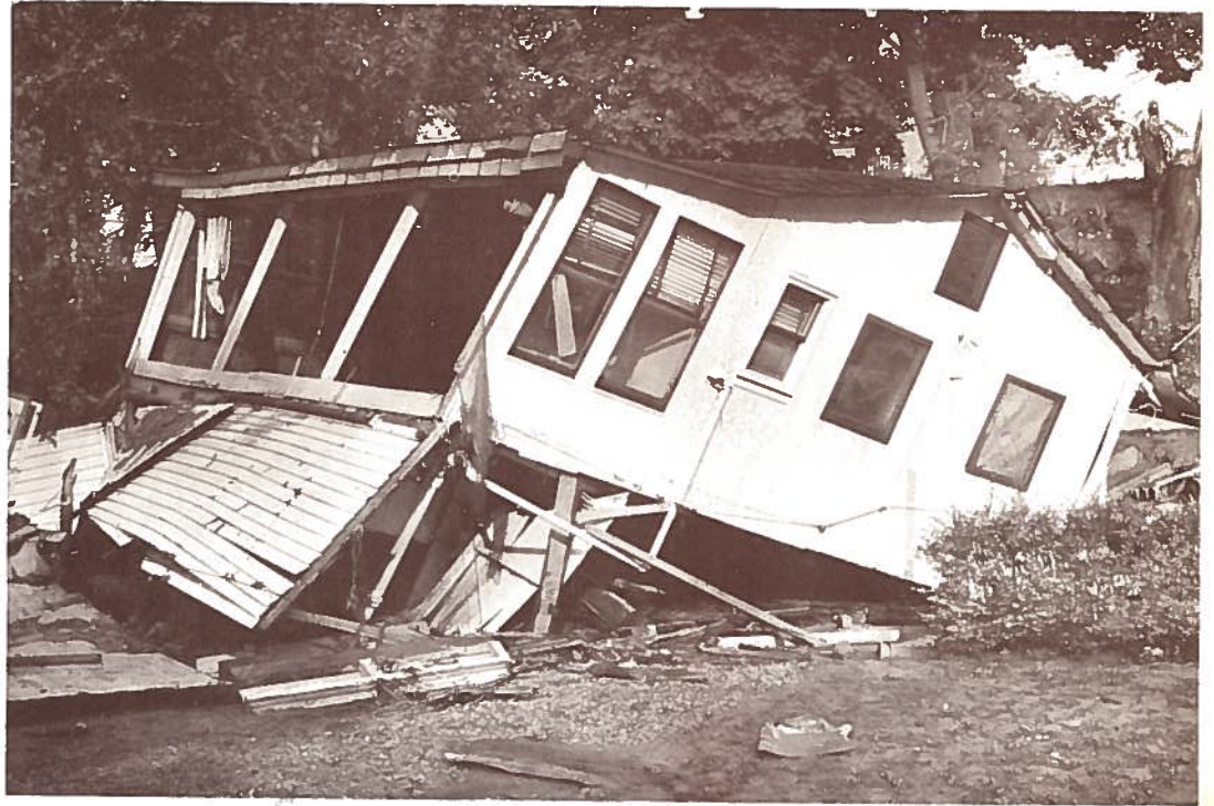
CAUGHT IN THE DELAWARE RIVER Narrows north of Easton, this bungalow was swept from its foundation by the flood.
