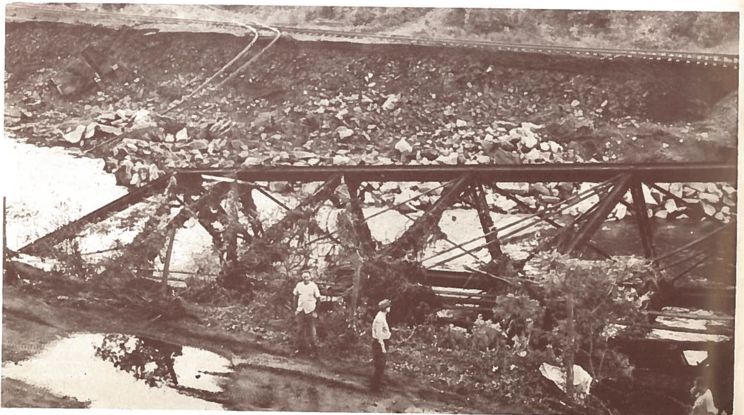
A LACKAWANNA RAILROAD BRIDGE at Scranton is flung into the Lackawanna River by the flood's fury.
