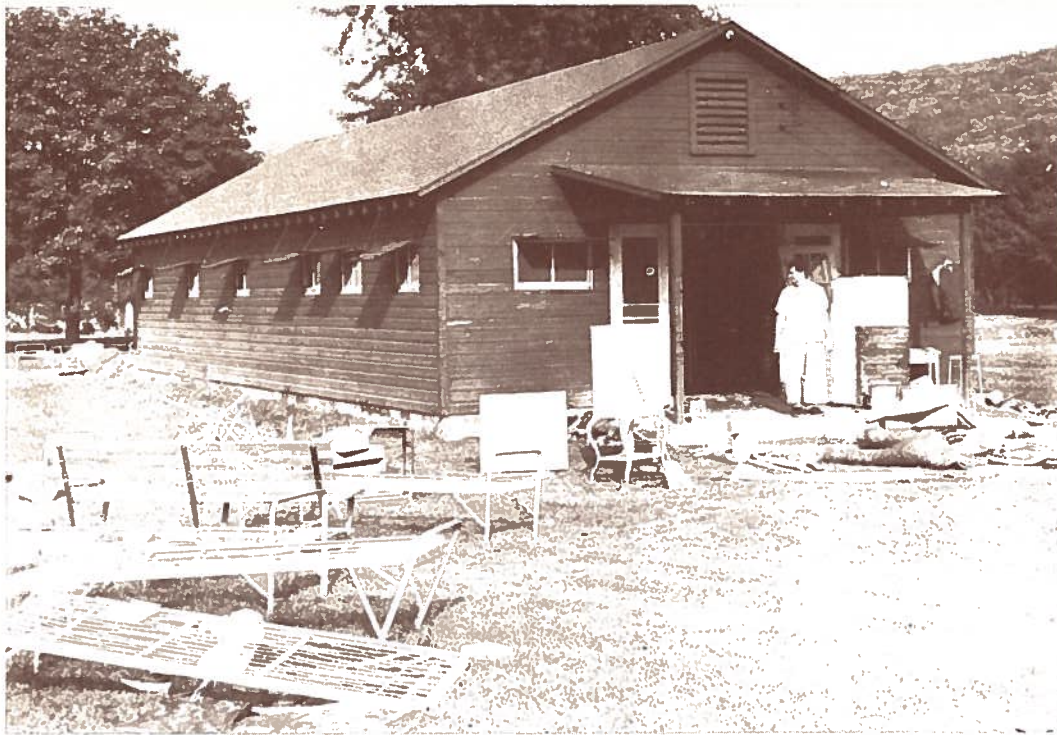
ABOVE IS ONE OF FEW BUILDINGS to escape wreckage at Camp Miller, 6 miles northeast of Minisink Hills, boys camp run by the Lutheran Ministerium of Pennsylvania. This is the infirmary which stood north of the wrecked mess hall.
