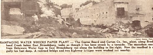
RAMPAGING WATER WRECKS PAPER PLANT — The Coates Board and Carton Co., Inc., plant, along Broad Creek below East Stroudsburg, looks as though it has been struck by a tornado from Delaware Water Gap to East Stroudsburg, ran along the building to the right. Now the roadbed is a gully ten feet deep. A railroad bridge and two highway bridges were washed out nearby.
