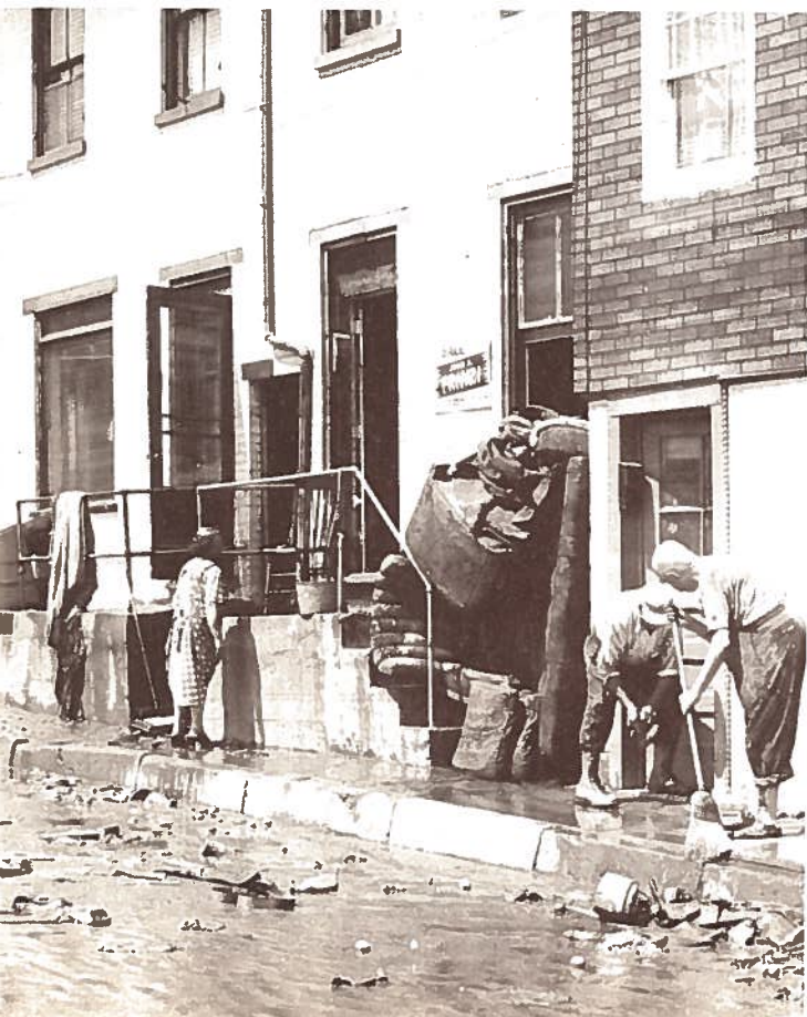
IN DOWNTOWN EASTON , just off South Third street, weary residents begin the work of restoration.
