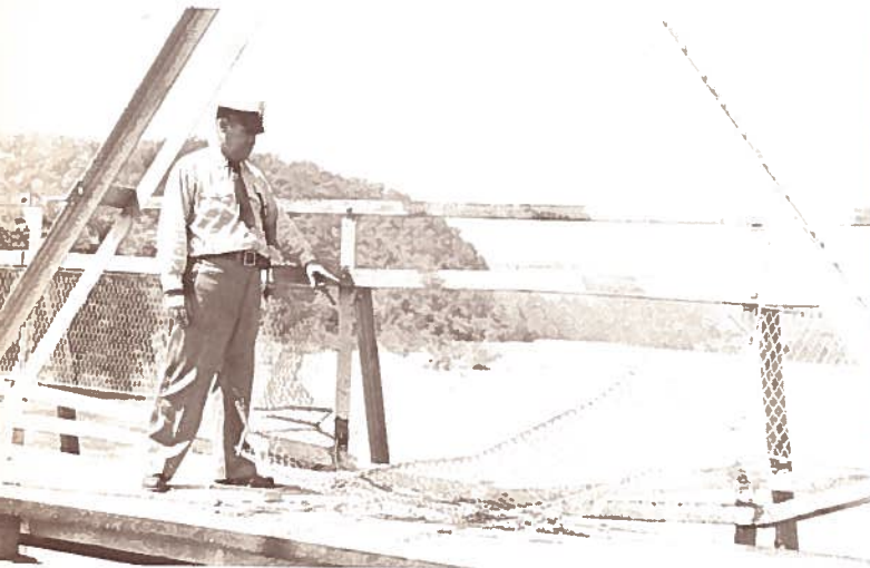
BRIDGE GUARD OF THE DELAWARE RIVER JOINT Toll Bridge Commission inspects a section of the free bridge at Belvidere, N. J., where the river's violence created damage.
