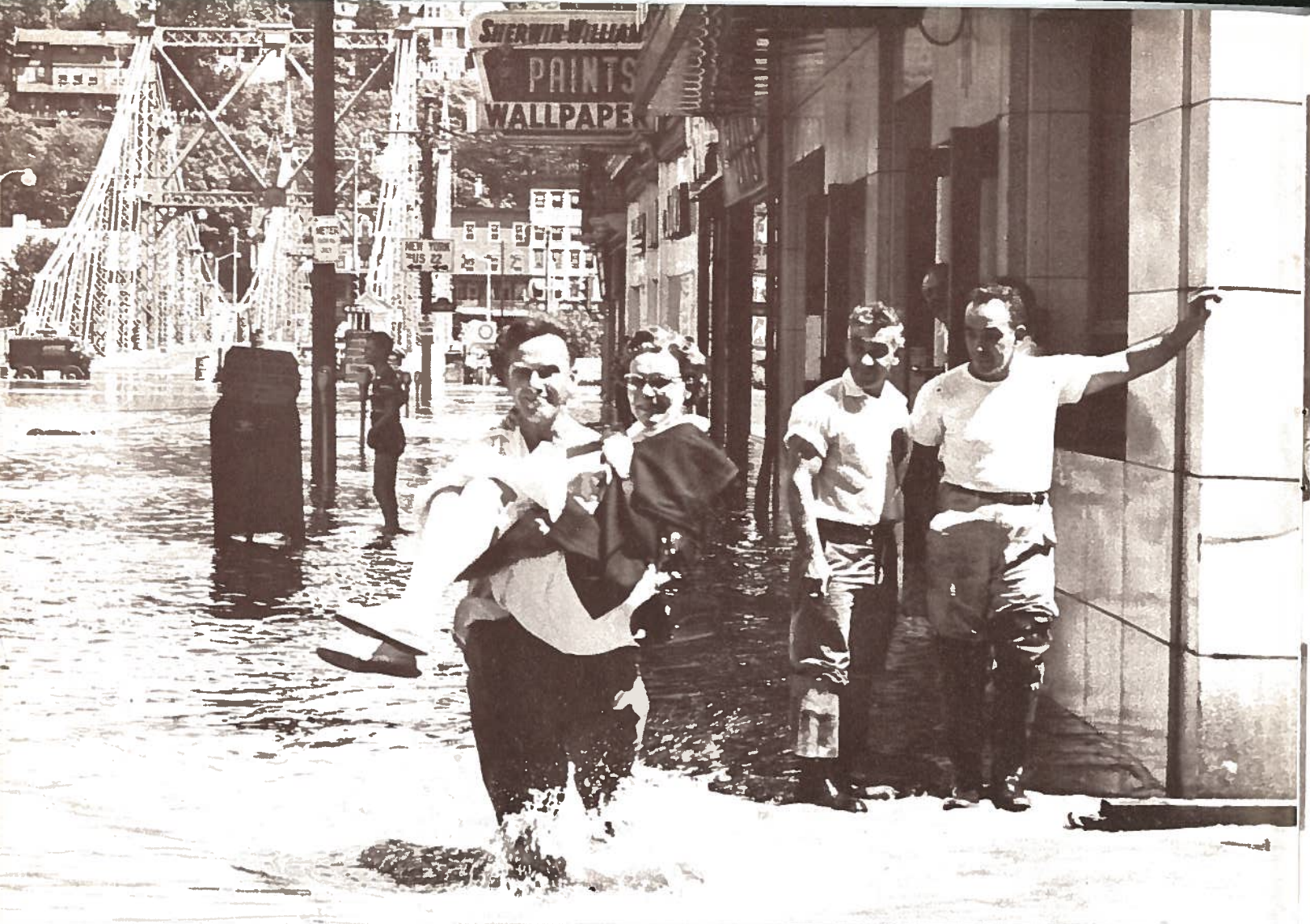
CHIVALRY IS WET but not quite dead as man gets feet soaked by the Delaware River, lady stays high and dry in muscle-power evacuation from the flooded area of Northampton Street, Easton.
