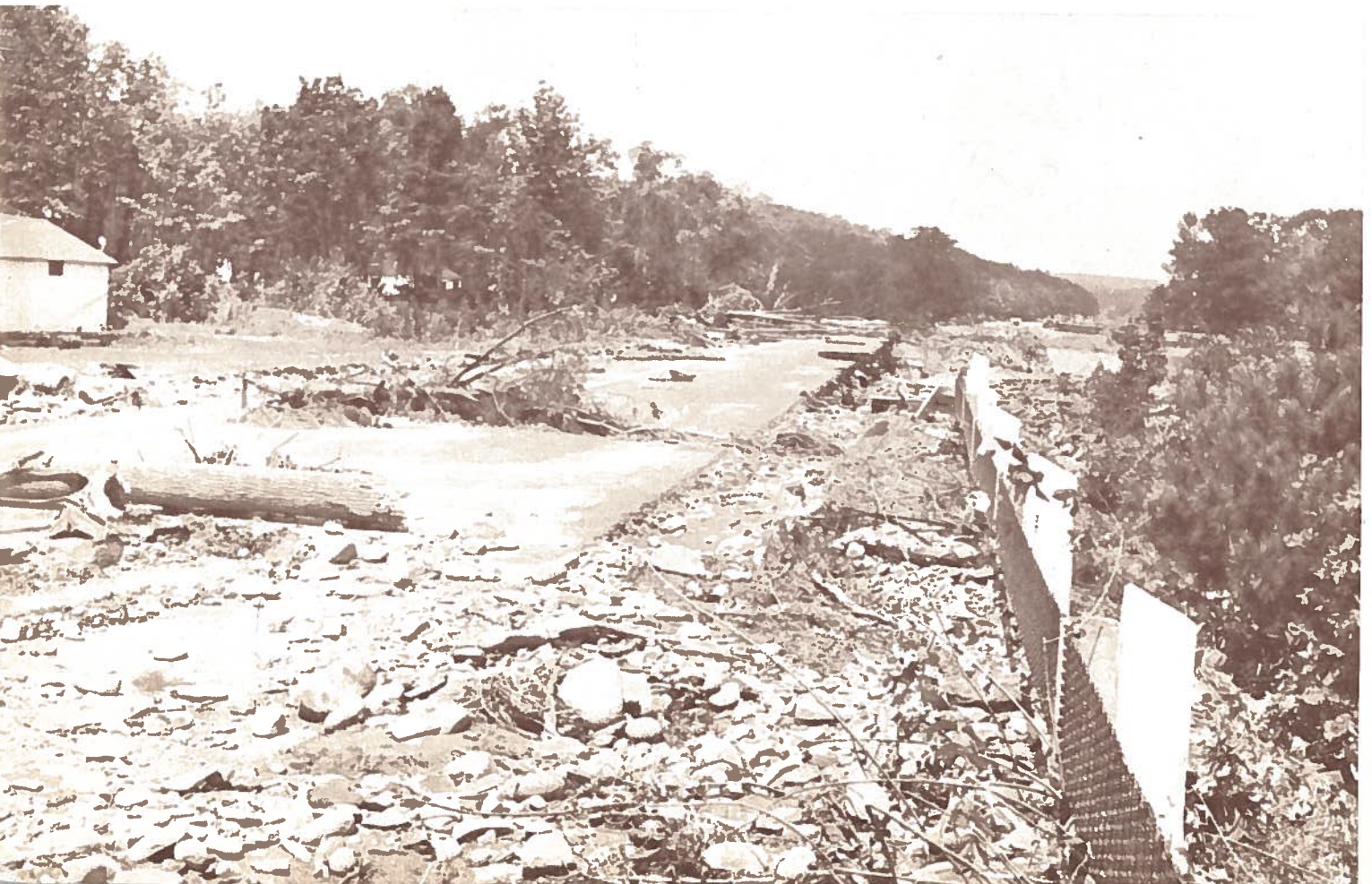
NEAR PENNBROOK CAMP along Route 90 in Monroe County where campers could look toward area in right of picture where Camp Davis was wiped out.
