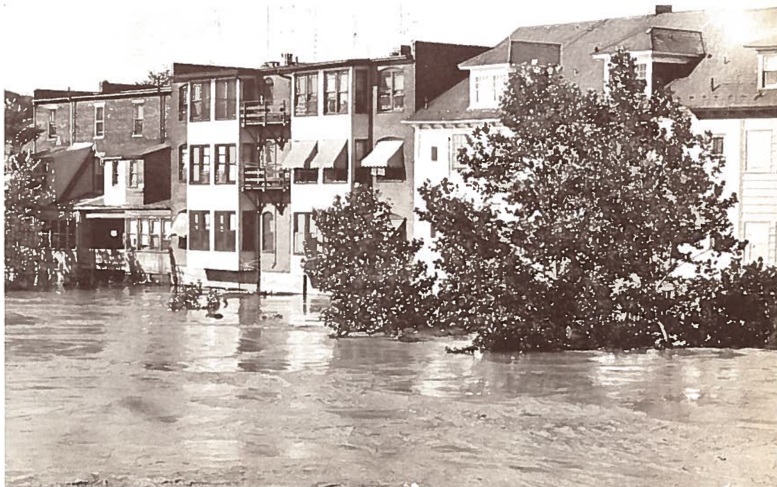
DAMP BACK YARDS — Flood waters swirl around the backs of homes on South Front street, Easton, along the Delaware.
