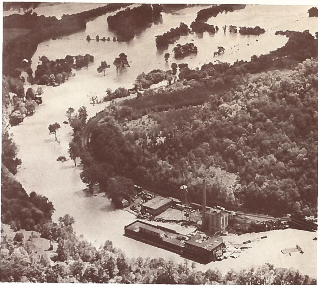
A PAPER MILL, A HIGHWAY BRIDGE and a railroad track are wrecked by rampaging Brodhead Creek near Minisink Hills.
