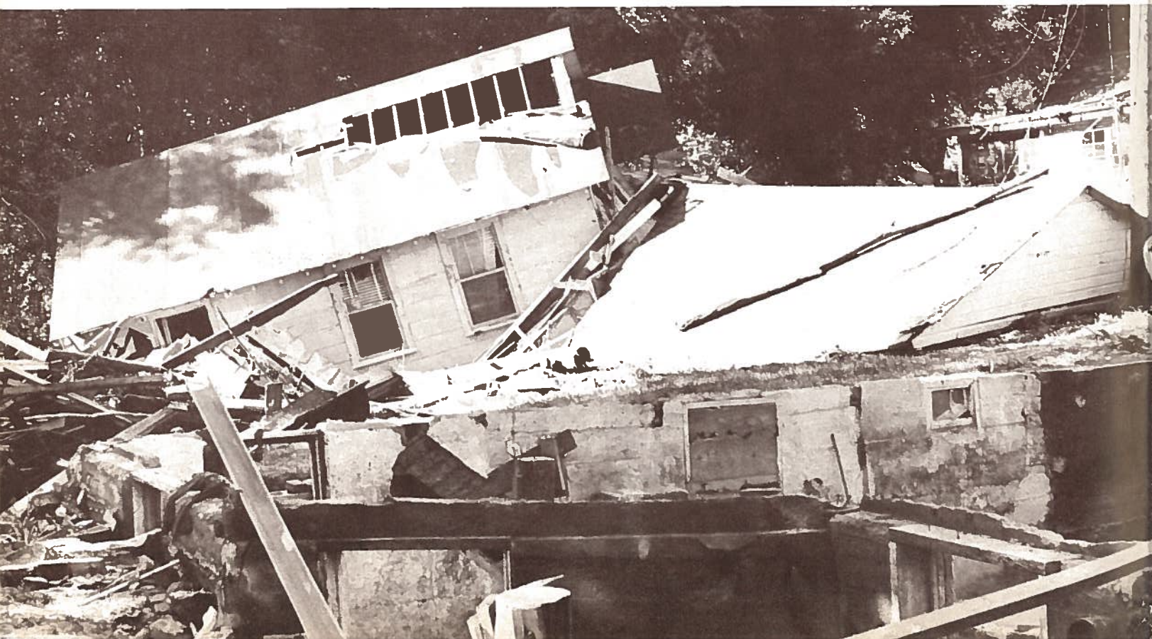
ONE AND ONE MAKE TWO , and two are entirely too many when the Delaware River uses its hurricane-fed force to combine two homes in one jumble of wreckage near Raubsville.
