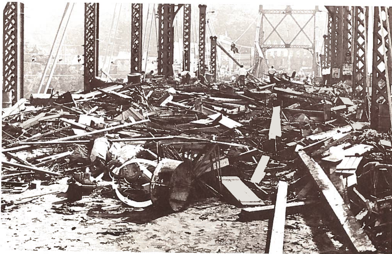
HORATIUS NEVER BLOCKED A BRIDGE more effectively than these tons of upriver debris on the free bridge over the Delaware between Easton, Pa., and Phillipsburg, N. J. And if you got past the debris, you found a hundred-foot section ripped out of the center span by the flood.
