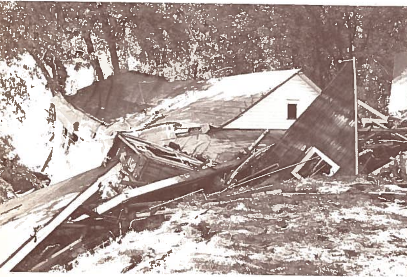
A CASUALTY OF THE JOINT FORCES of the Delaware River and the picturesque Delaware Canal near Raubsville, Pa.
