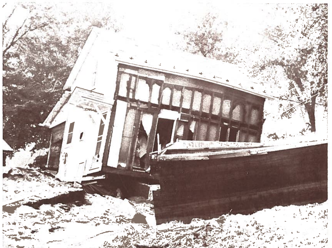
A HOUSE AT CARPENTERSVILLE tips crazily after the flood.
