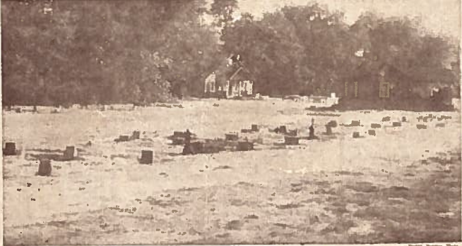
The Lutheran Camp northeast of Shawnee was ravaged by the Delaware River. About 200 boys were led to higher ground in human chain through waist-deep water Friday.
