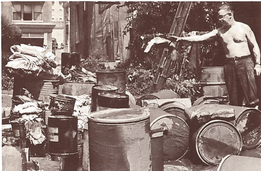
BARRELS, ROLLED OUT — After the flood, work begins in Hull's Court, Easton.
