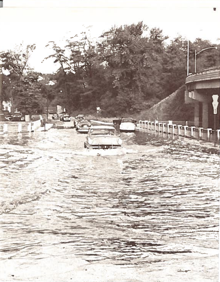
TRAFFIC PLOWS THROUGH DEEP WATER on the bridge spanning Bushkill Creek at the junction of Bushkill street, Pearl street, and Bushkill drive in Easton.
