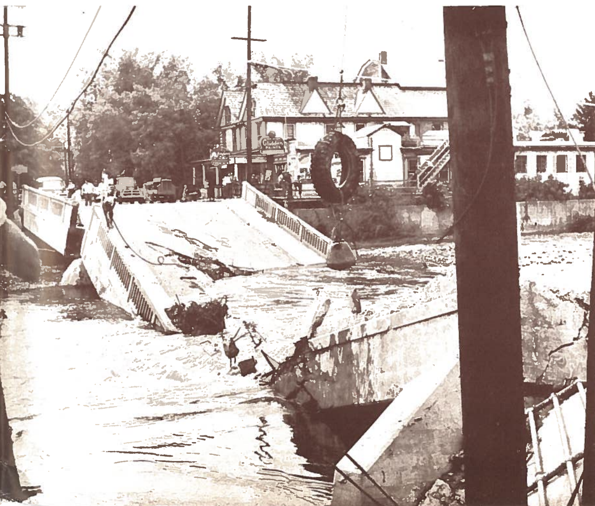
WORKMEN breaking up a bridge west of the center of Stroudsburg on Route 209.
