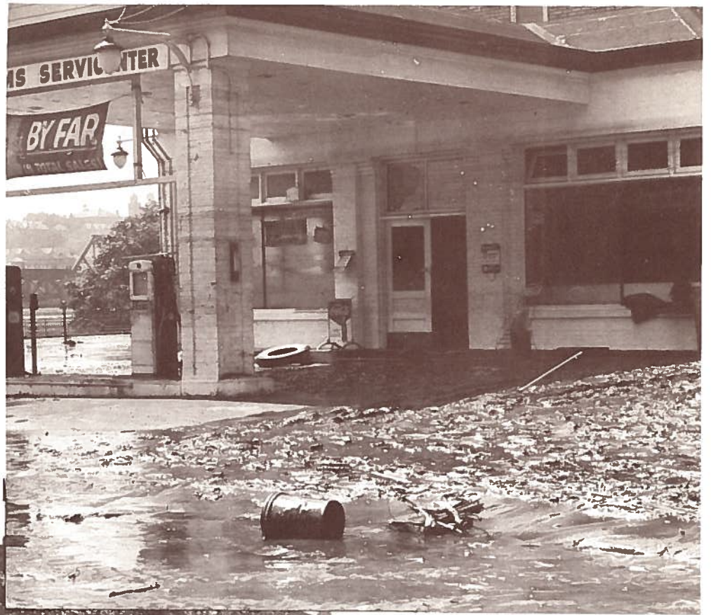
MUD OOZES ACROSS THE CONCRETE at the service station across from Scott Park in Easton.
