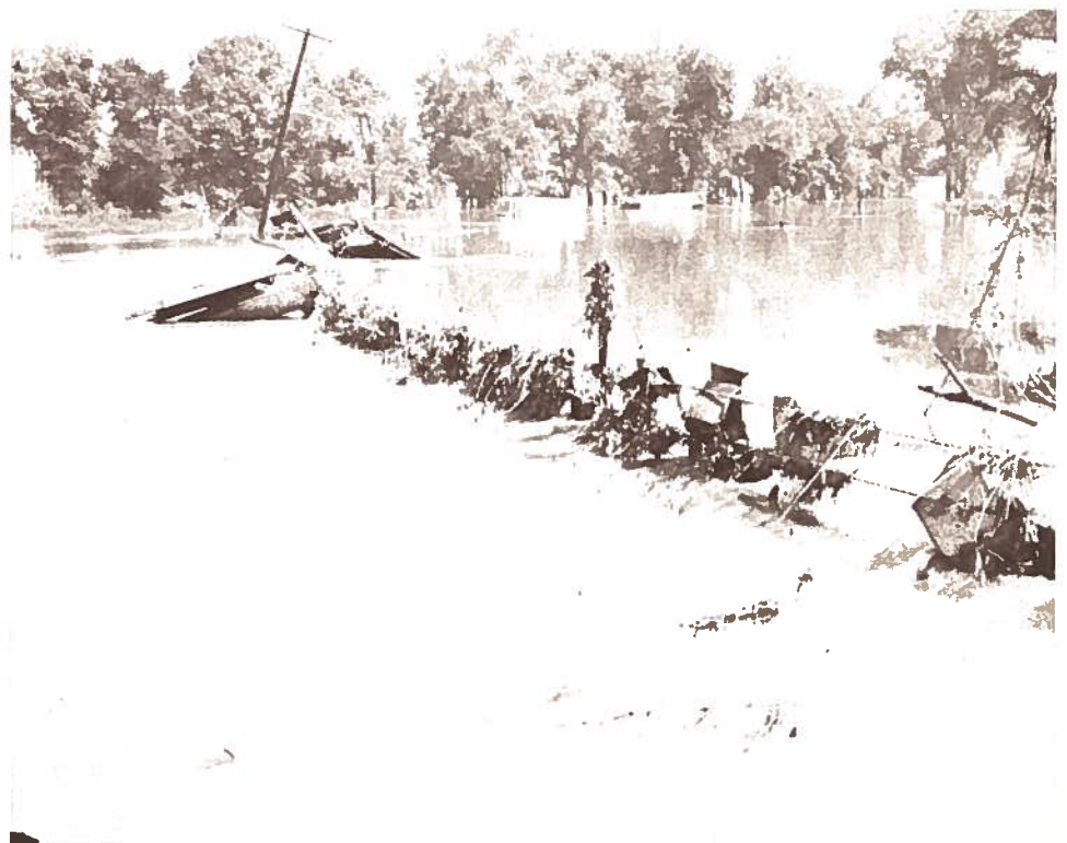
THE BEGINNING AND THE END of Rt. 46 near Manunka Chunk is marked by this debris-festooned guard rail. Trucks are marooned on the highway in the distance.
