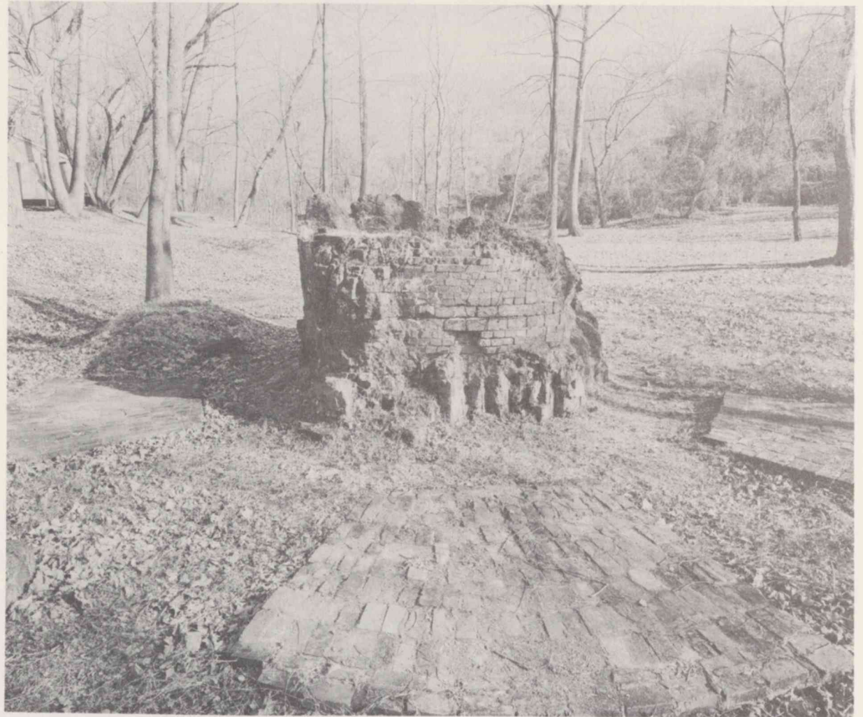
Glendon Iron Company ruins in Hugh Moore Park, along the eastern section of the Lehigh Canal. All that appears to remain of this once-successful industry are the deteriorating foundations of three blast furnaces built between 1844 and 1850. Public appreciation of the site's historic significance could be enhanced by making interpretive information available on an adjacent marker.
