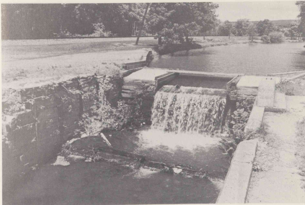
A—2. Photo 8. Lock 10 spillway, near Weissport.
