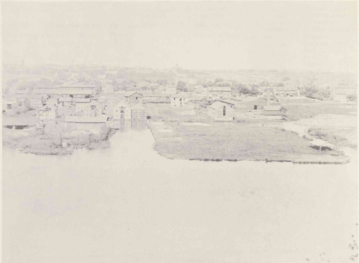
View of Allentown showing the boat basin and early industrial sites along a slackwater section of the canal. Courtesy of the Lehigh County Historical Society.
