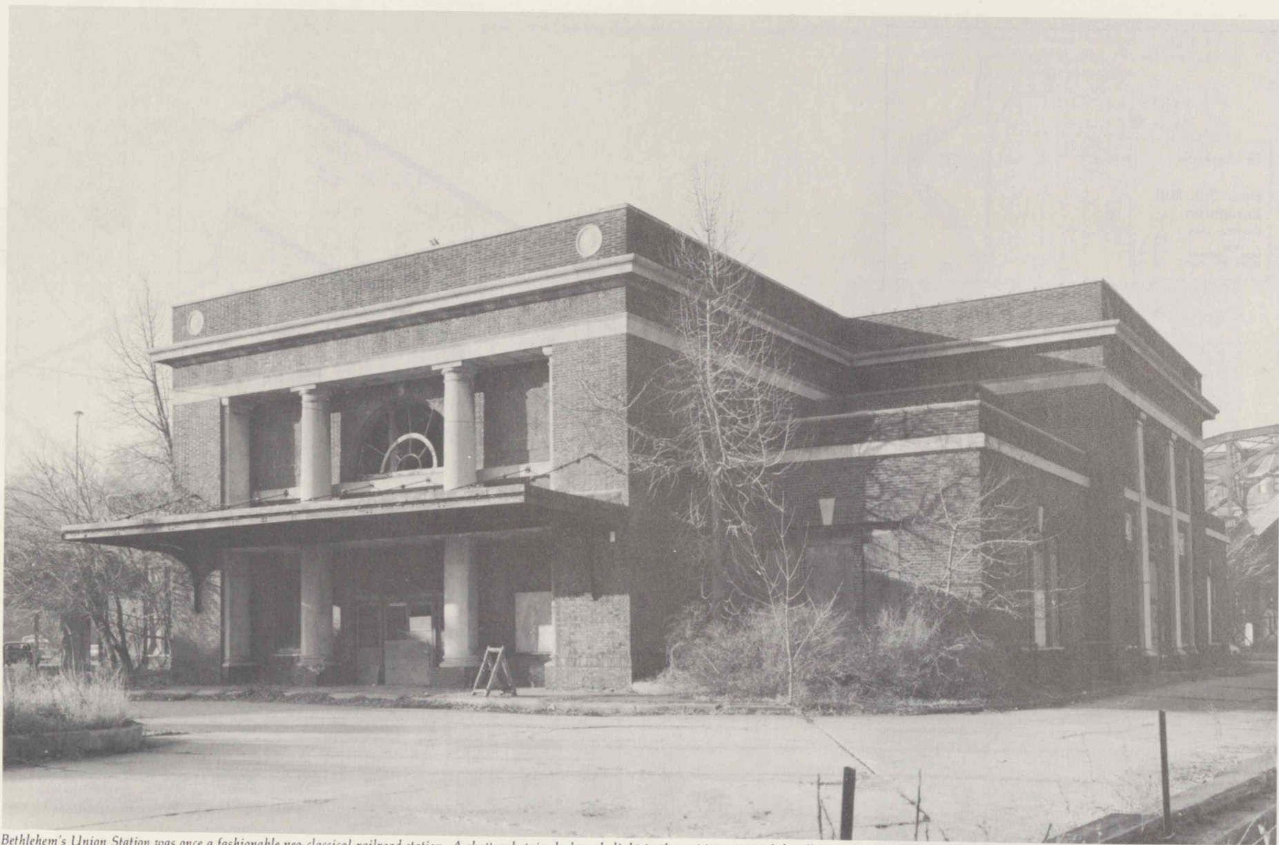
Bethlehem's Union Station was once a fashionable neo-classical railroad station. A shattered stained-glass skylight in the waiting room, tiled walls, remains of waiting benches, and cast-iron fences and railings are reminders of its former elegance. It was constructed in 1924 to serve the Lehigh Valley Railroad and the Reading Railroad. An underground corridor, now blocked, connected the station interior with the tracks outside.
