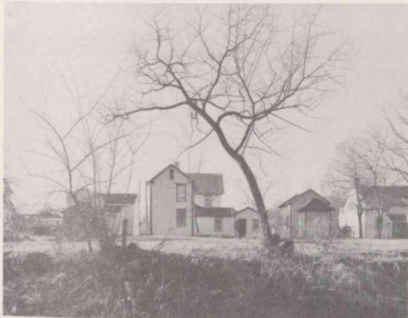
Freemansburg's Main Street runs parallel to the canal. The canal is the backyard for many of the nineteenth century residences along the street.
