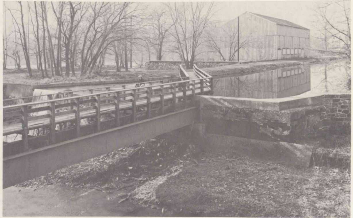
Monocacy Creek Aqueduct, looking west toward the canal.
