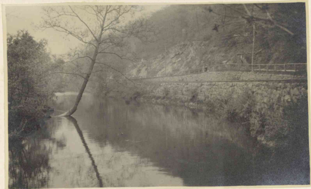
View upstream , From bridge.
