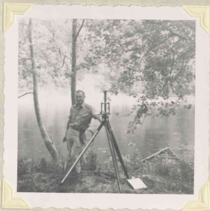
Set-up on center line of dam, New Jersey side, opposite exposed ledge rock on Pennsylvania side of river.
