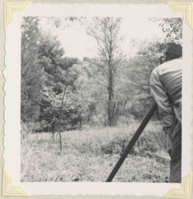
Carrying center line of dam through heavy brush and trees.
