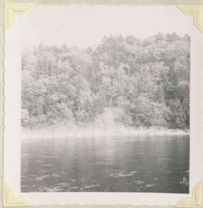
Exposed ledge rock on Pennsylvania side which would form tie-in of abutment..
