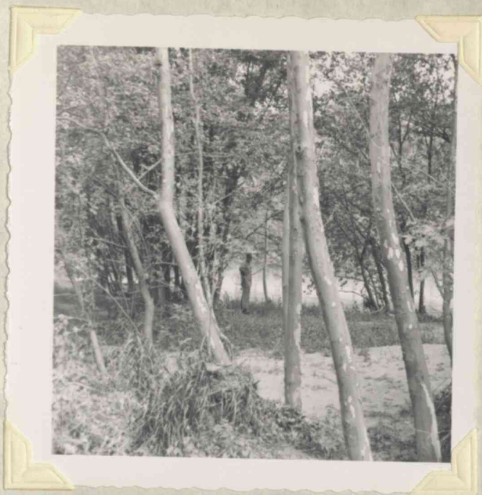
Establishing line to edge of river at proposed site of dam..
